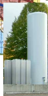
LNG storage (liquefied natural gas) to be used as a back up for biogas
