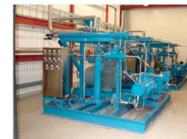
Two high pressure compressors with 100% redundancy
