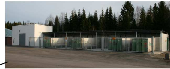
Filling station for movable gas storages for the supply of biogas to public filling stations
