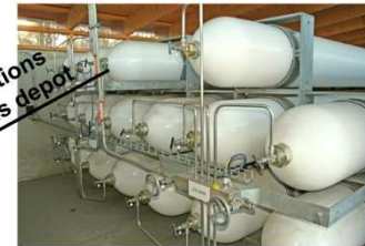
Gas storage divided into three sections. Maximum pressure 350 bar and capacity app. 6000 Nm 3
